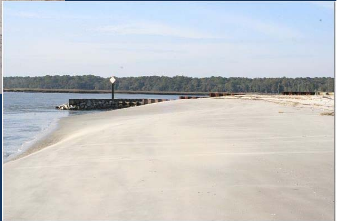
6 Mth Post-Construction (stable)
