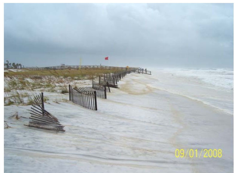
Figure 2 Runup, overwash and erosion from Hurricane Gustav along the eastern end of Pensacola Beach, FL (Escambia County R-149).
