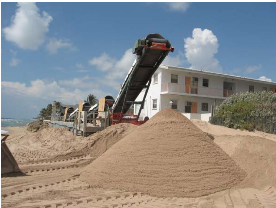
Conveyor systems placing sand on the beach
