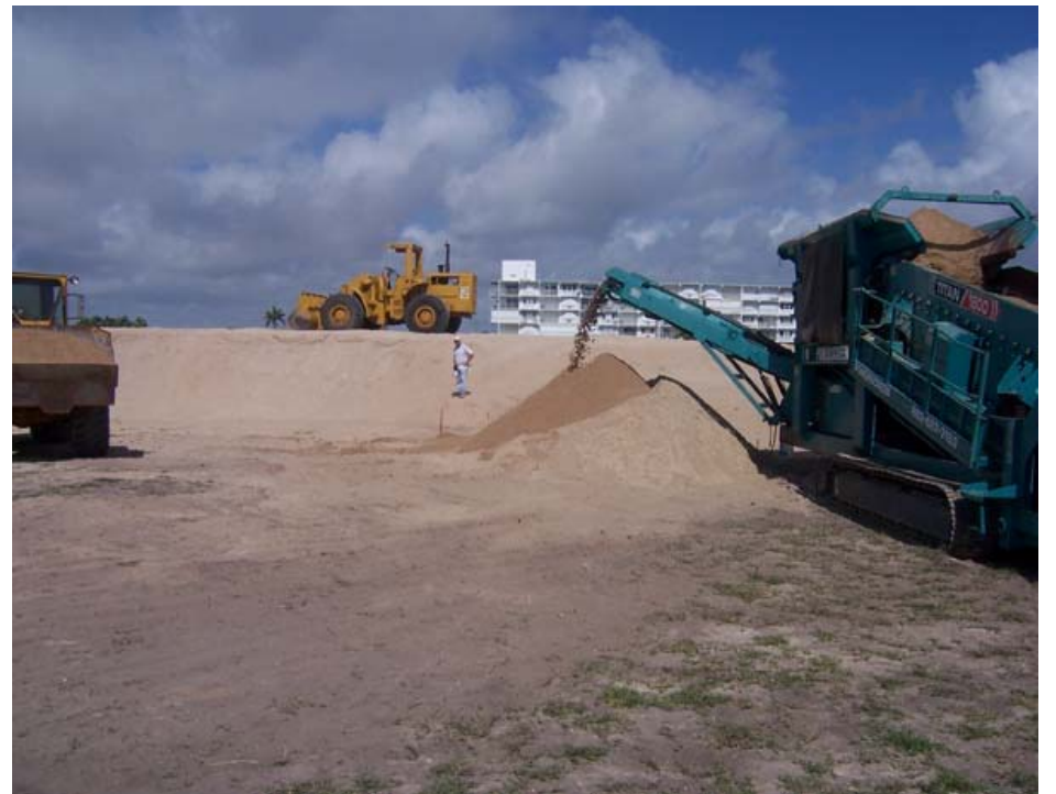
Sand screening operation for material to place on the beach
