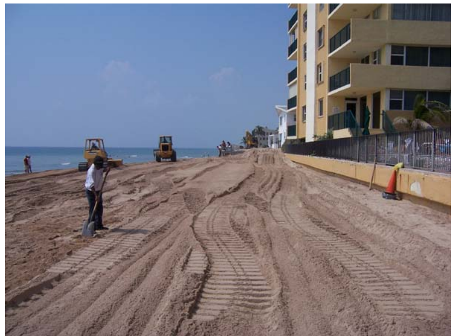
Final grading of project
