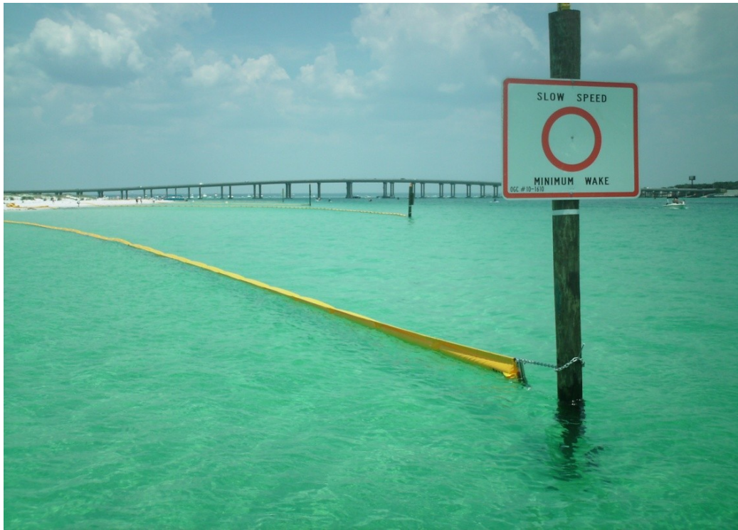
Figure 6. First boom successfully installed in the pass by CPE team.
