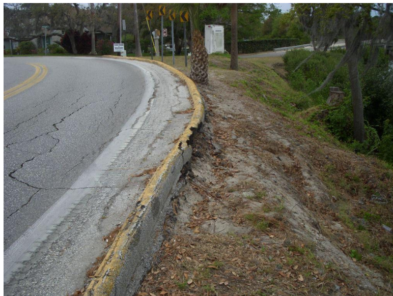
Existing Conditions along the south segment of Kreamer Bayou.
