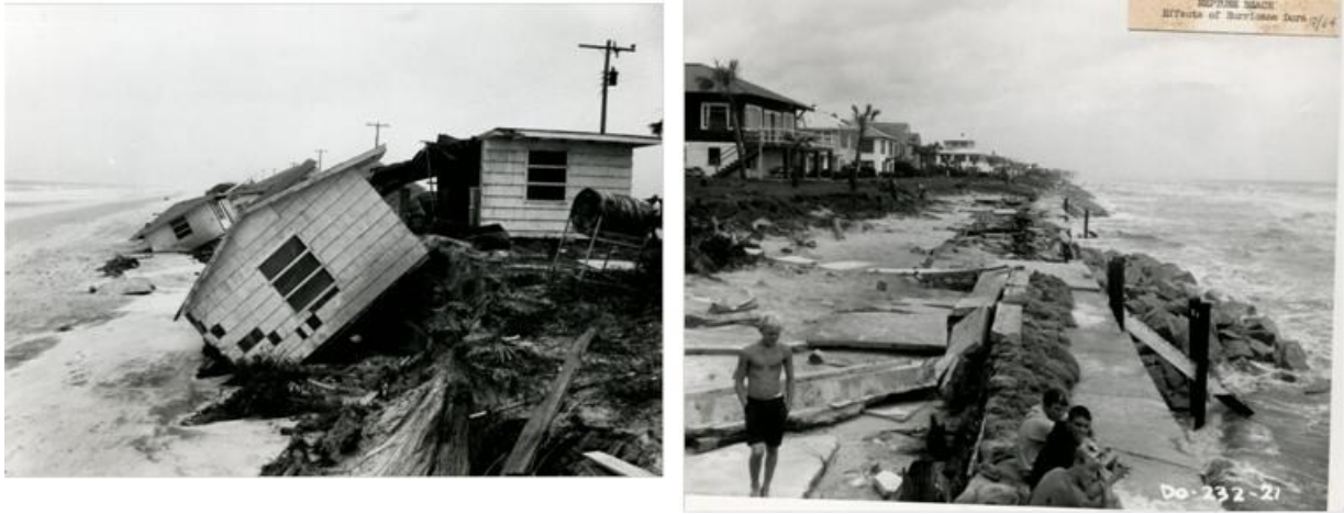
Figure F: Typical storm damage from the 1962 nor'easter and Hurricane Dora, 1964.
