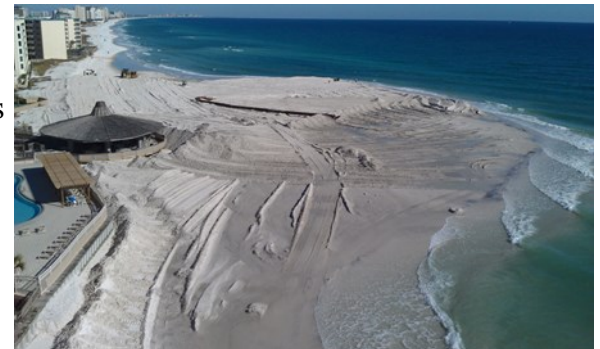
Photograph of the Western Destin Beach Restoration Project taken February 2, 2013, courtesy of Taylor Engineering
