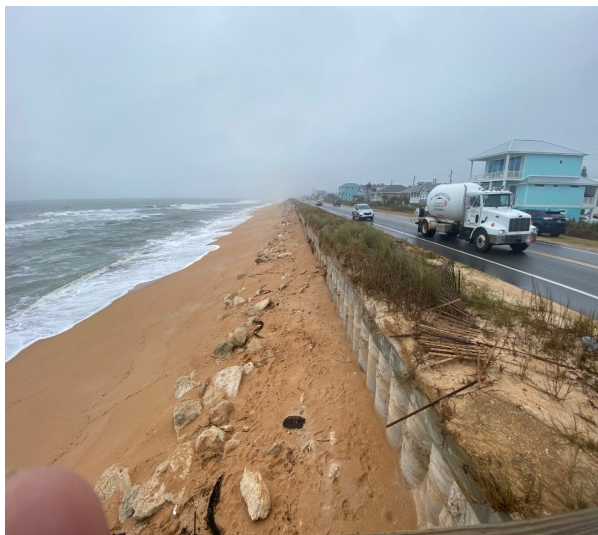
Figure 9: Scour from Hurricane Nicole exposing 3.5-foot to 10-foot height at face of buried secant-pile bulkhead/seawall (source: Lead author's photo).
