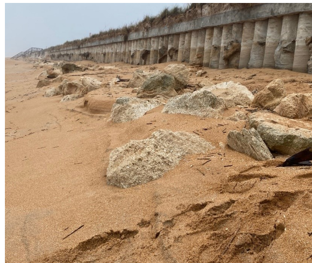
Figure 9: Scour from Hurricane Nicole exposing 3.5-foot to 10-foot height at face of buried secant-pile bulkhead/seawall (source: Lead author's photo).
