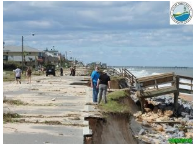
Area hard hit by Hurricane Matthew, photo courtesy of FDEP
