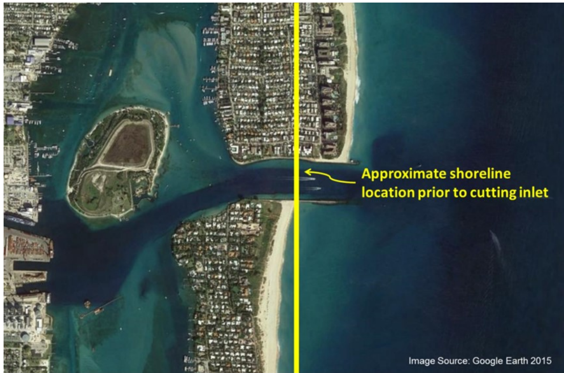
Figure 2. Shoreline offset at the Port of Palm Beach entrance (recreated from Dean, 2007).
