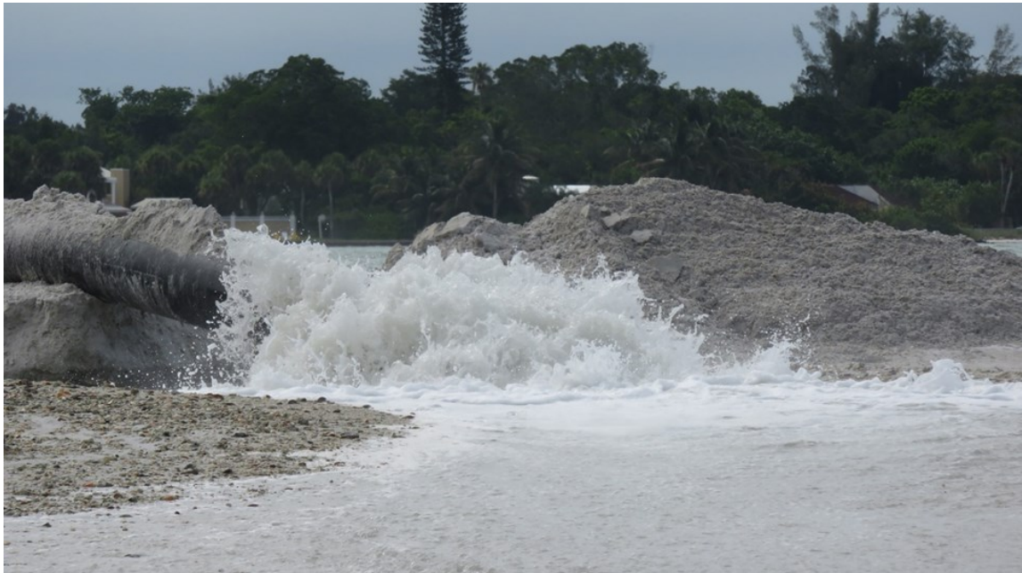
Figure 1: Sand being pumped onto Lido Key, Sarasota during construction in 2020.
