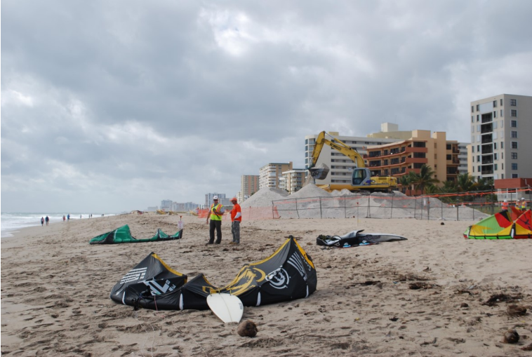
Photo courtesy of USACE Jacksonville District Broward Segment II, Post-Sandy, 1-16-14
