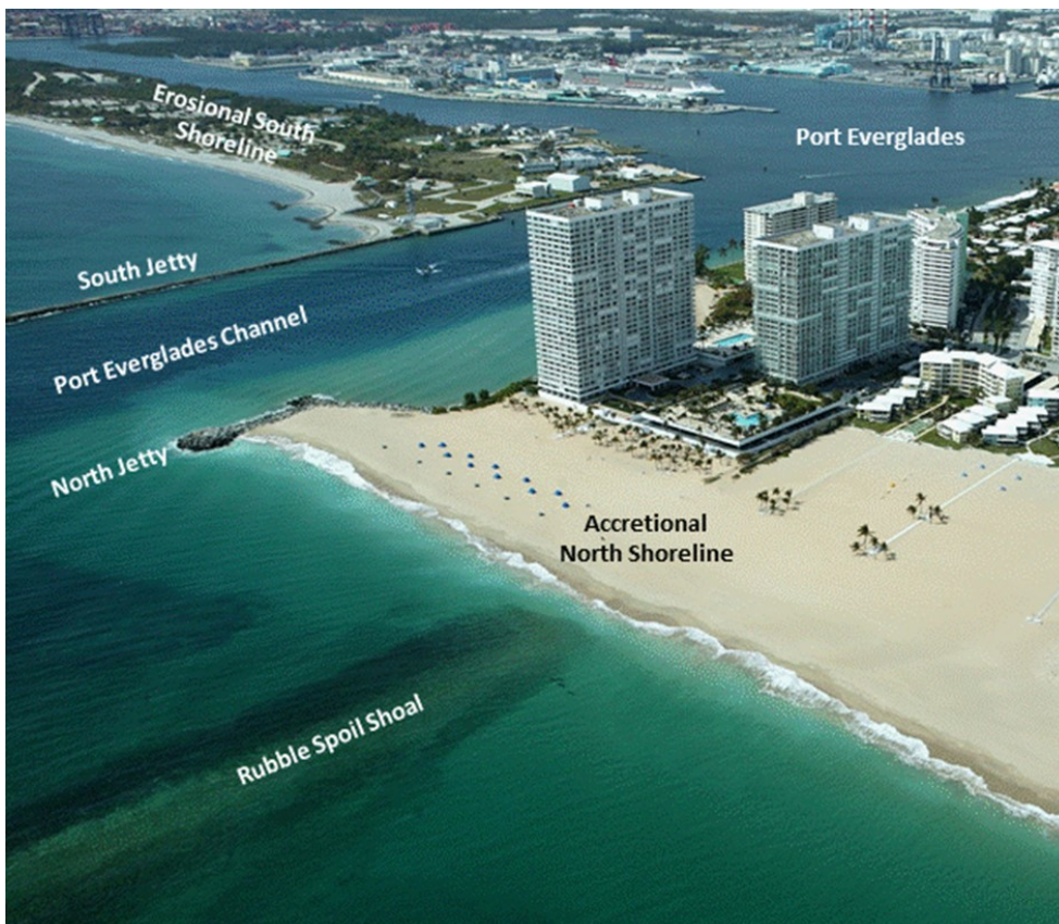
Existing configuration of inlet and adjacent shorelines, looking southward.
