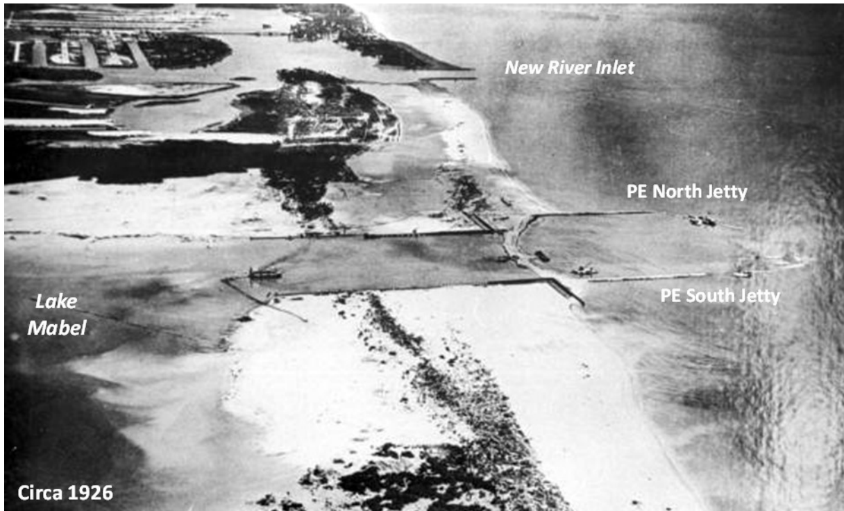
Photo taken in 1926 of inlet construction activities at Port Everglades. In this photo, the New River Inlet in its open condition appears at the top center. Port Everglades Inlet, under construction, is seen in the center of the photo. At this time, the bund separating the Atlantic Ocean and interior waters at Port Everglades was still in place.
