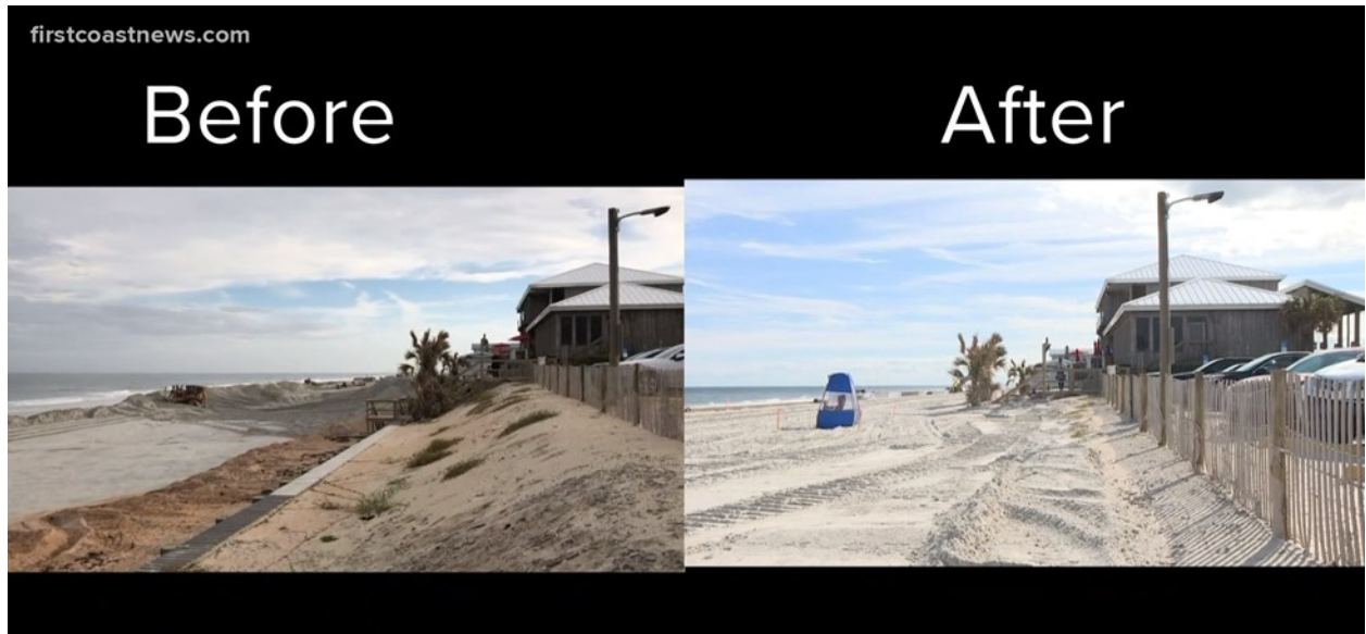
Figure 2: Before and after photos at Reef Restaurant in Vilano Beach (photo courtesy of firstcoastnews.com)
