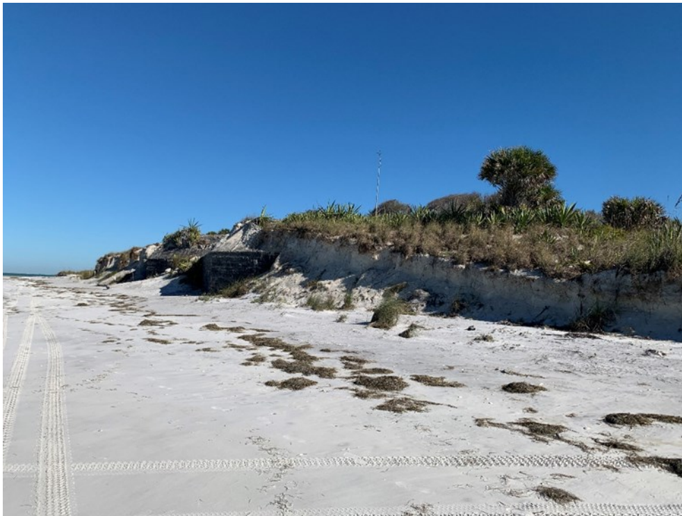
Photo looking north along west shoreline of Egmont Key in January 2022. Note Battery McIntosh exposed on beach.
