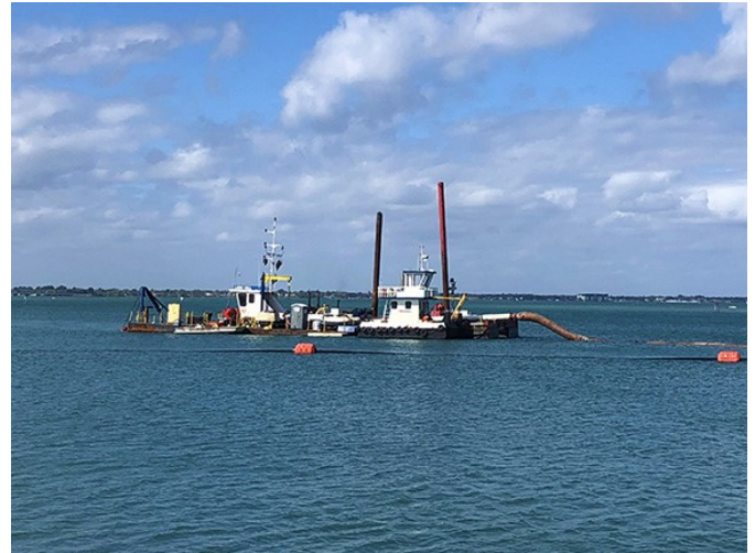
Ferreira Dredge over trap
