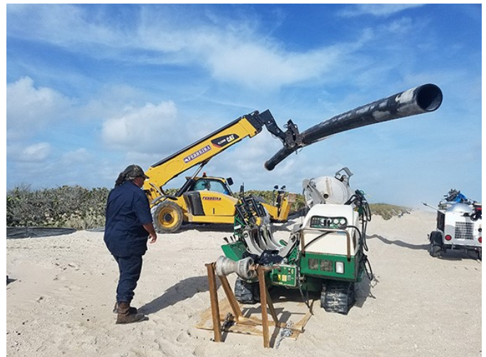
Ferreira fusing pipe at R-8
