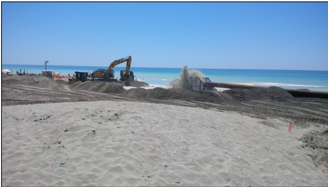
Beach nourishment work taking place on Venice Beach in Sarasota County
