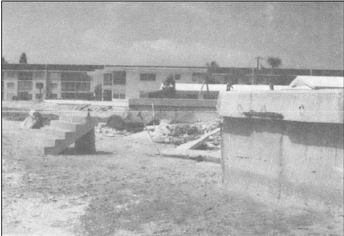
Concrete seawall in Venice Beach destroyed by a storm in 1982
