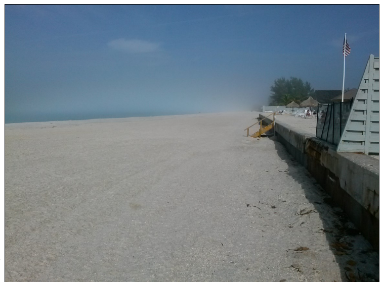
January 6, 2014, Construction just completed. Funded as part of the Corps of Engineers 2012 storm recovery efforts along with the State and County cost-sharing.
