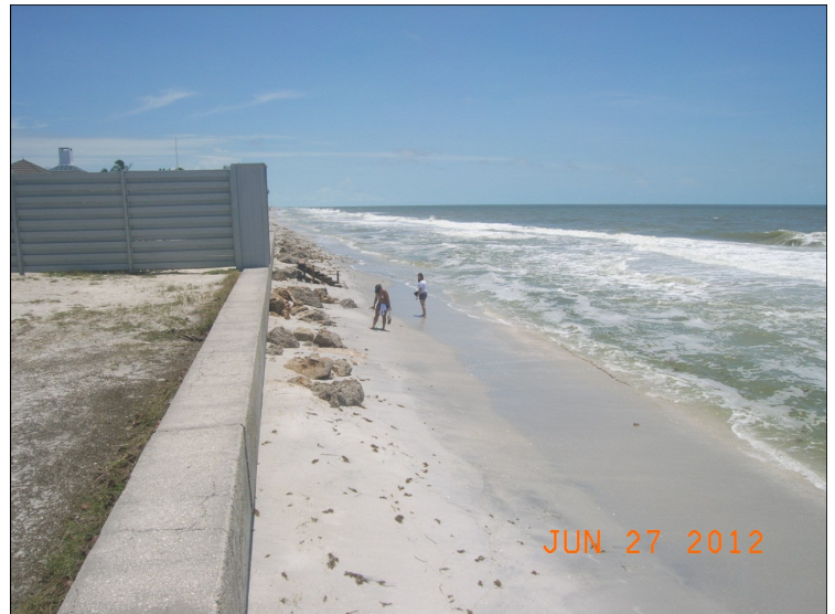
Lee County's Gasparilla Island federally-authorized beach project, Post Tropical Storm Debby.
