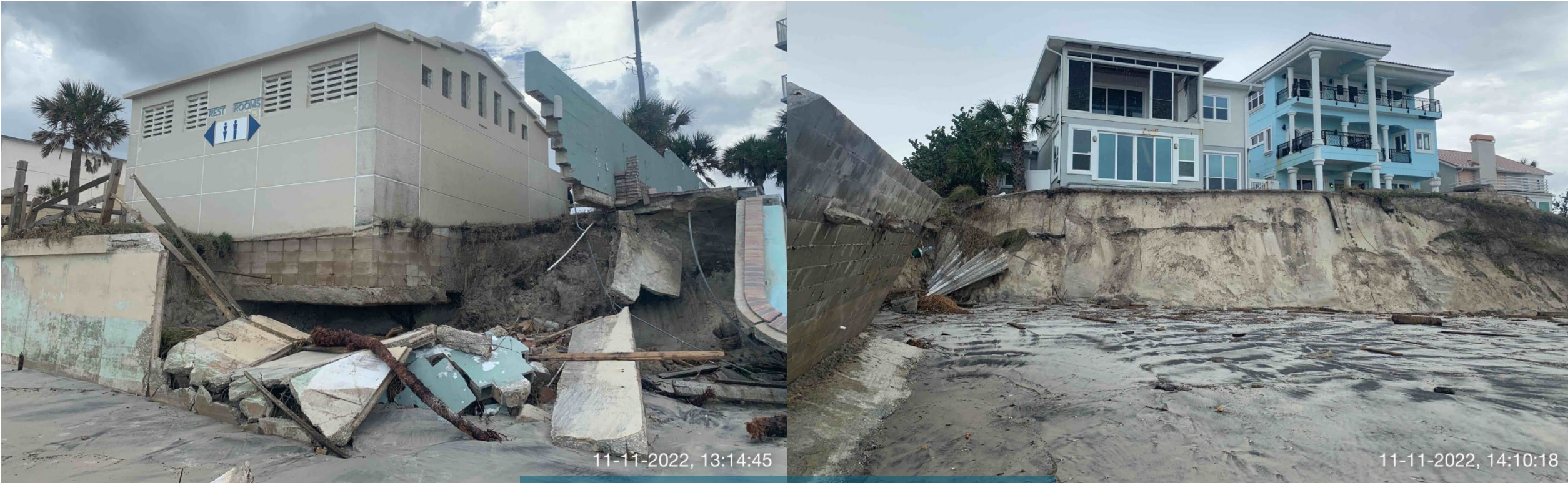
Hurricane Nicole Damage (Volusia County, 2022)
