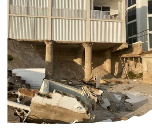
Buildings in danger of collapse with inadequate foundations for the open coast
