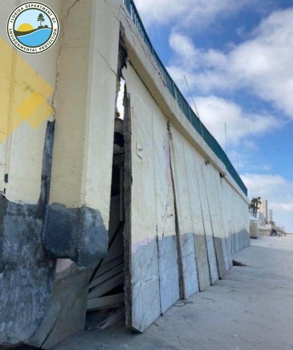
Inadequate sheet pile penetration & corroded reinforcing steel
