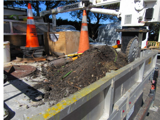
Source: Andy Holland, City of Naples 10 Filters @ GSB & Park Shore Dr ~1 CY (1,000 lbs) Annual Cleanout
