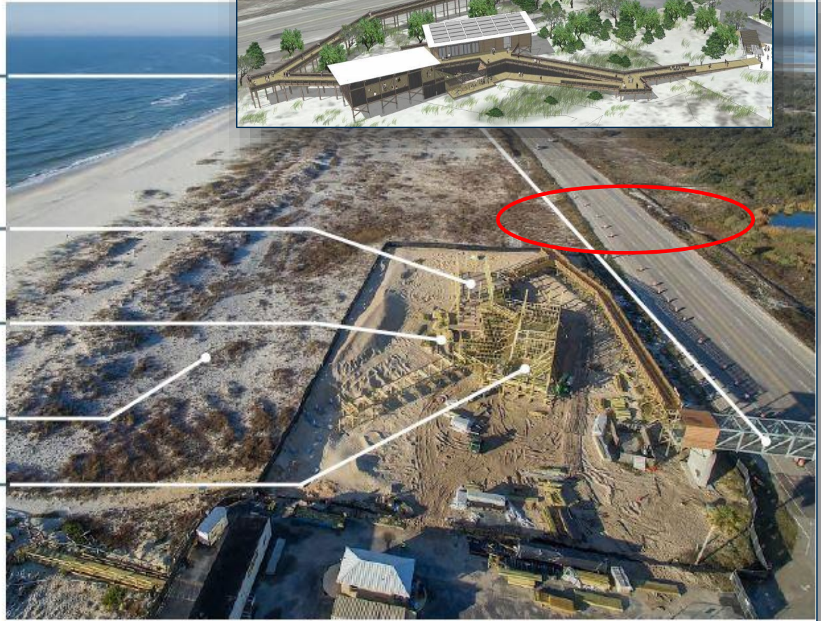
Interpretive Center Construction Progress - Dec 2017
