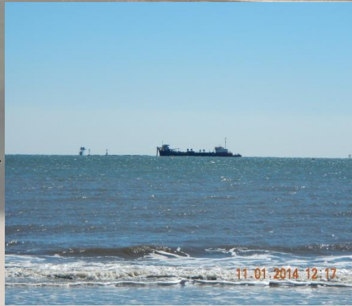
Hopper Dredge Pump to Fill Area
