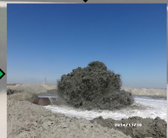
Discharge at Fill Area
