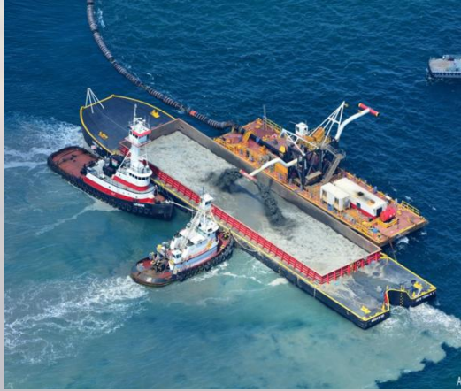
Cutterhead Dredge Excavation and Filling Scow Barge via Spider Barge
