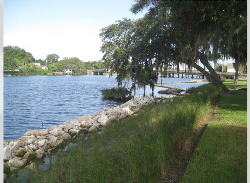
Riverside Garden Park Shoreline Stabilization, Tampa
