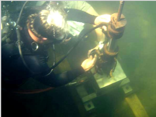
Underwater Anchor Installation
